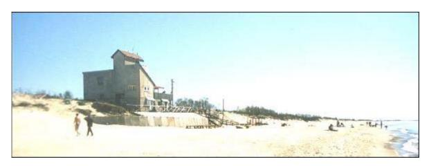
*Fig. 3: Melnrage rescue station and leisure facilities with the exposed concrete revetment on the retreating beach. Photo: E. Paplauskis, May 2001.*
